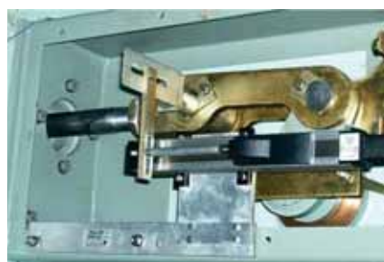
Actual pictures of Transducers mounted with their fixtures
